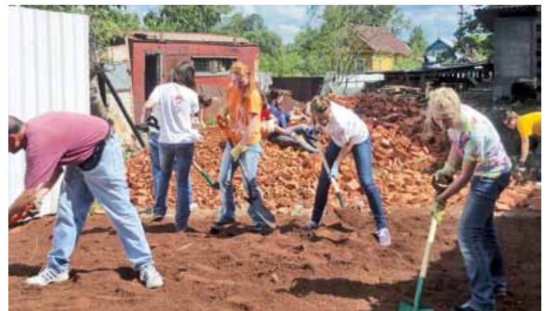
Moving sand and gravel.
